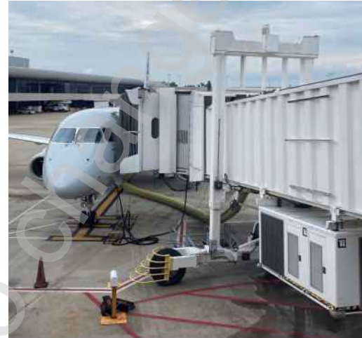
Ground Power Unit (GPU) at Gate 43
